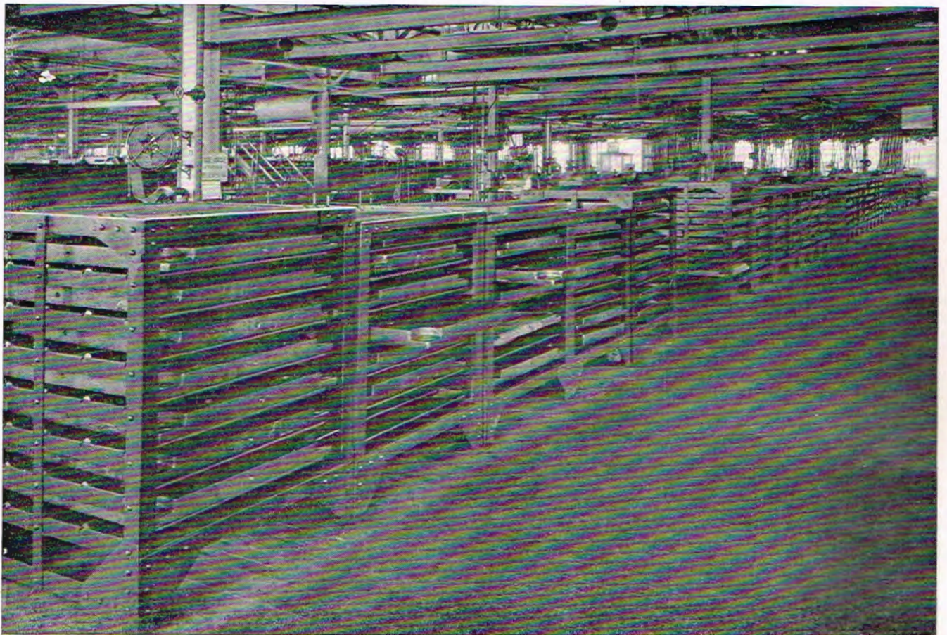
Thirty steel racks contain 210 special butt plates weighing 1,000 pounds each. These are a part of the tool equipment
