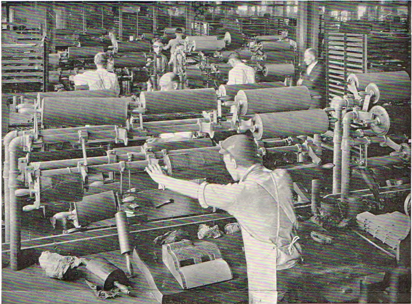
A section of the graining room
