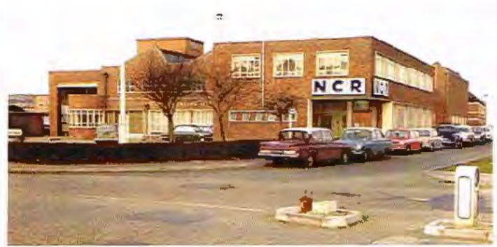
The Printing Division plant at Elstree is equipped with 34 presses.
