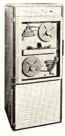
This high speed paper tape reader reads computer files at the rate of 400 or 600 numeric characters per second — eight or twelve times as fast as the desk top reader. All the file data needed to generate a fully automatic payroll can be stored on a single tape reel.
